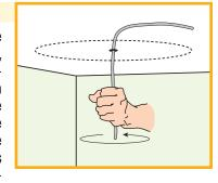
tion area as possible. Mark the center of the ceiling ring **(L)**, drill a hole and insert piece of wire bent at a 90 degree angle. Rotate the wire around 360 degrees. While rotating, feel for resistance that could indicate wire runs or other obstructions.
