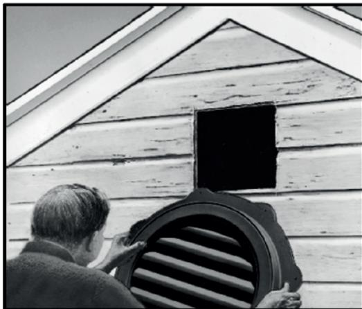
\* Rough opening refers to the minimum amount of unobstructed wall opening needed to maintain the Net Free Area.
