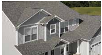
ROOFING AND VENTILATION
