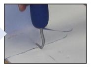
**Immediately** check seam by running testing probe along seam edge.
