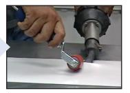
Use flat end of seam tester to tamp and hold down T-joints.
